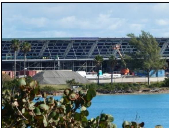
New airport under construction in January 2019
