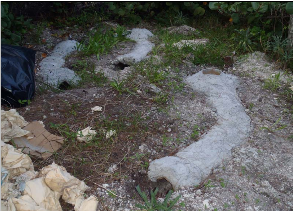
Fig. 9: New concrete Cahow nest burrows being built at “B” translocation site.
