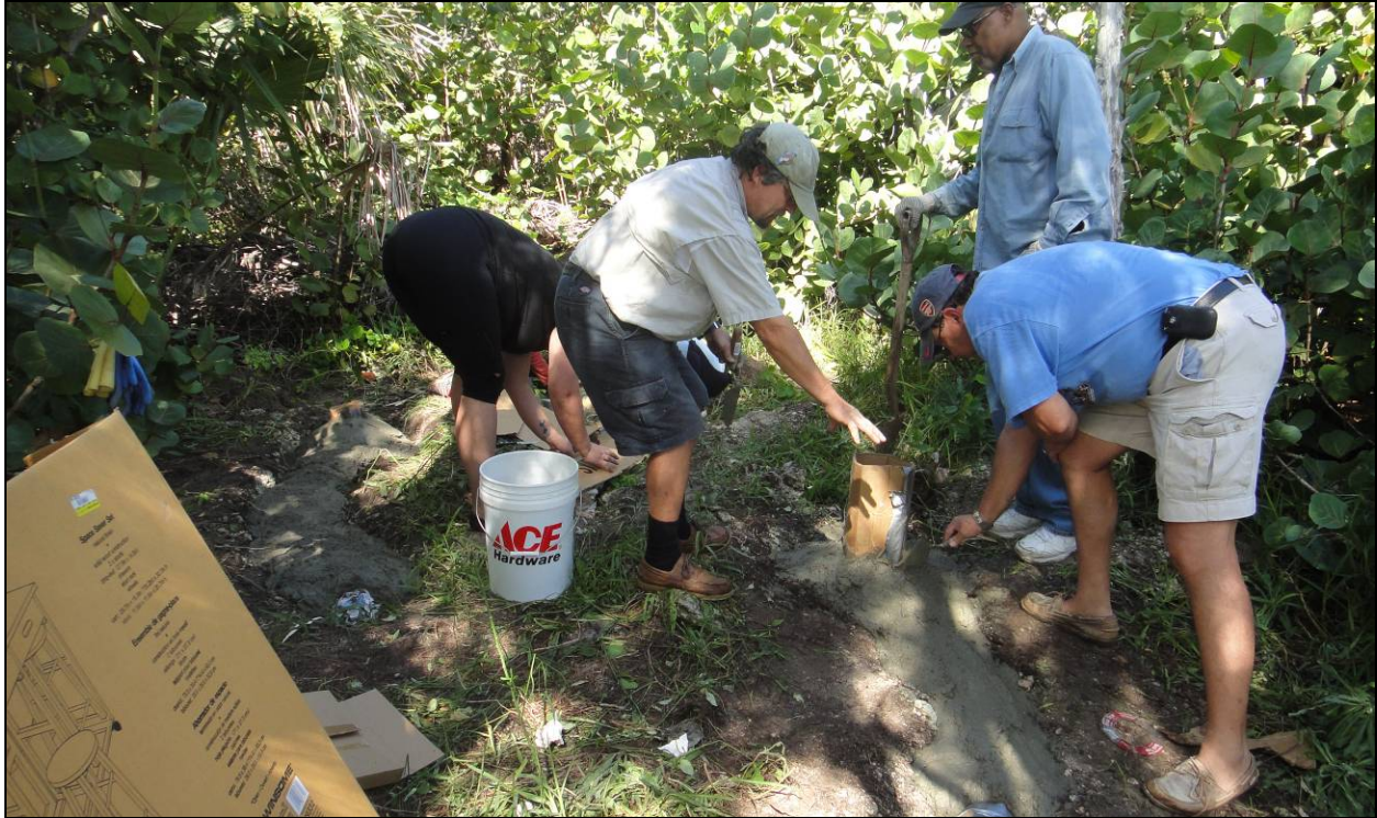
Fig.10: Ascendant volunteers working with Conservation Officer to build new concrete Cahow nest burrows at “B” translocation site.
