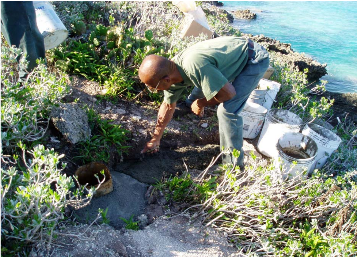
Fig. 3: Artificial Cahow nest burrows being constructed on Horn Rock
